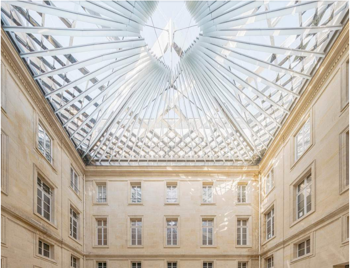
Verrière Hôtel de la Marine, Paris - Agence 2BDM et Hugh Dutton Associés/HDA © Nicolas Trouillard Executed using grade Aperam 304L with Uginox Meca 7D (Mirror polish)
