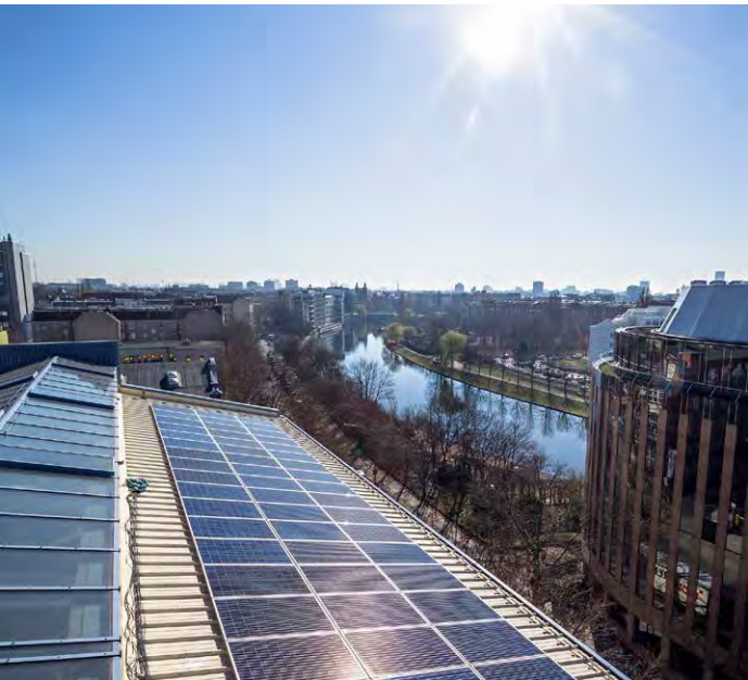
GSG Solar PV, Berlin, Germany
