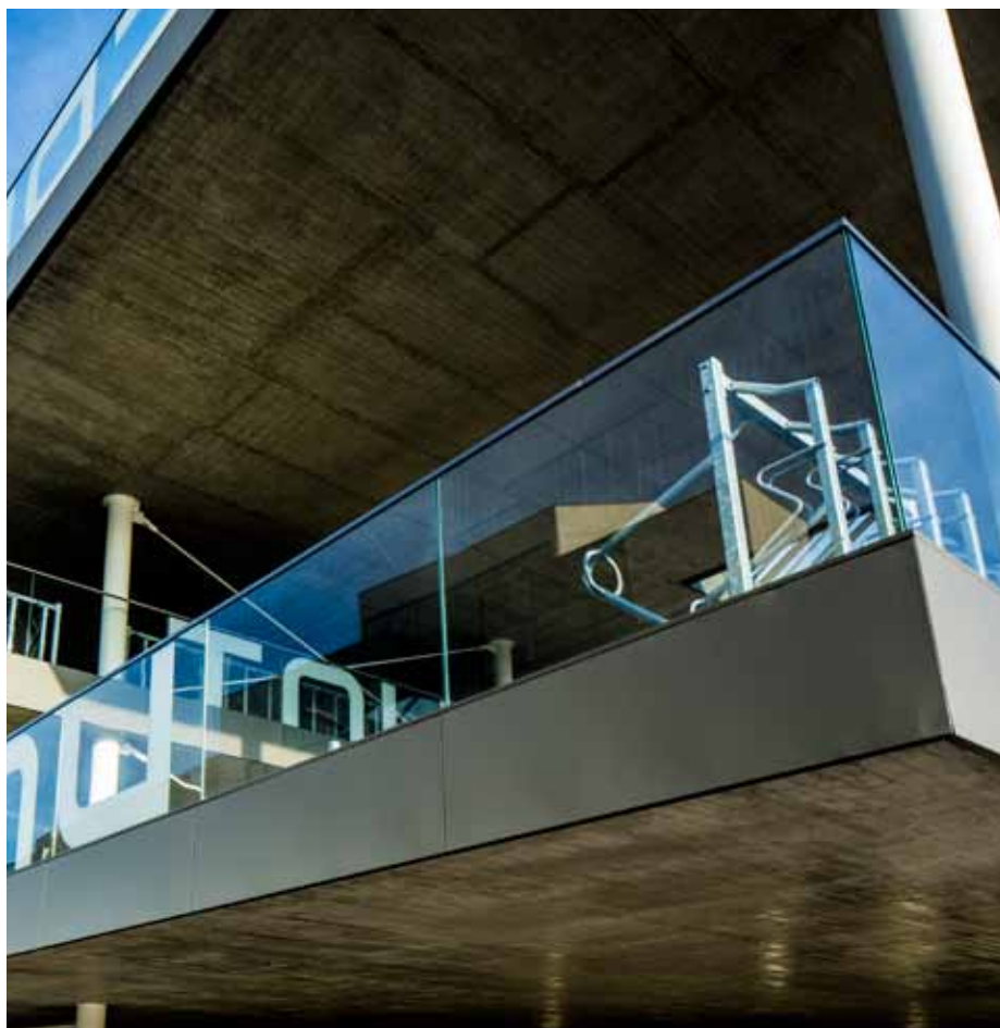
Bicycle parking facilities - Berchem railway station
