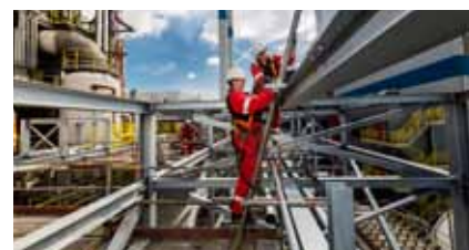
Scaffolding works at AVR (Rotterdam)
