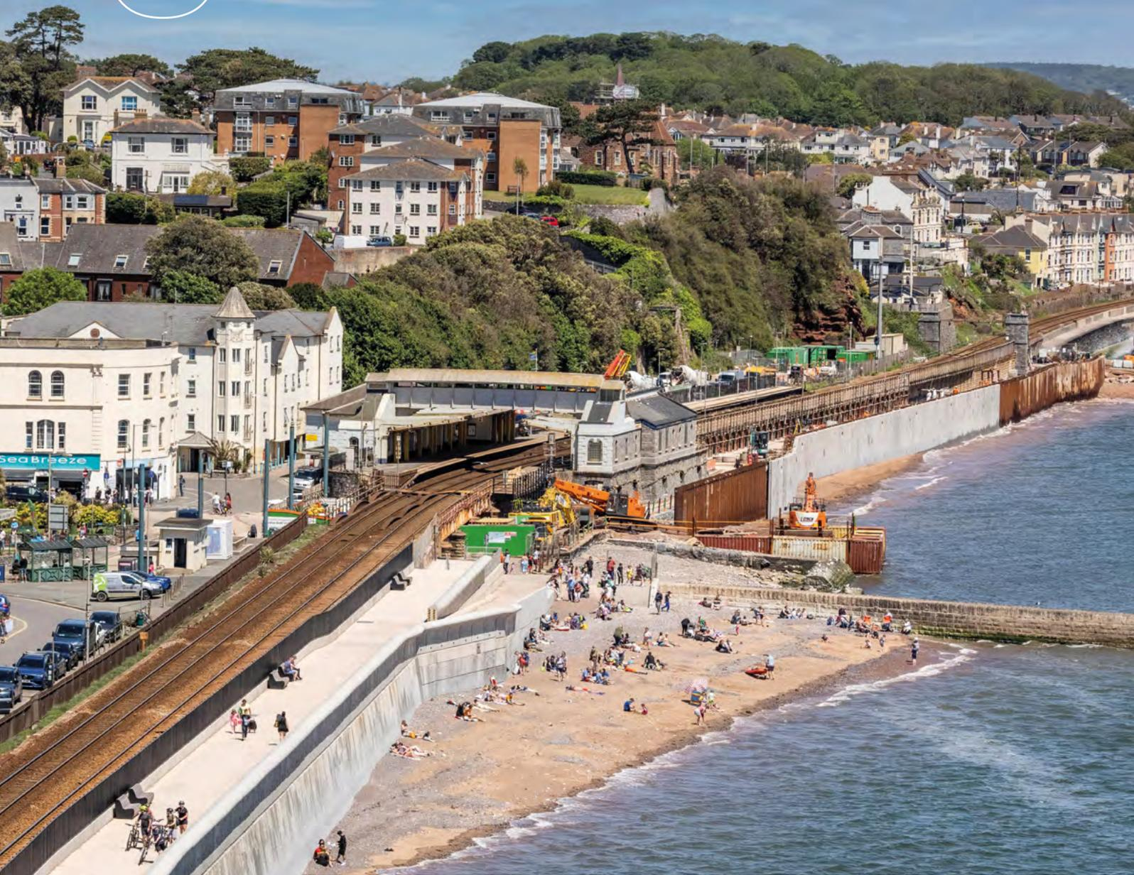
*The Dawlish Sea wall protects the railway line through the installation of panels, pre-cast blocks and recurve units for Network Rail. It will provide better protection against rising sea levels and extreme weather conditions for generations to come.*
