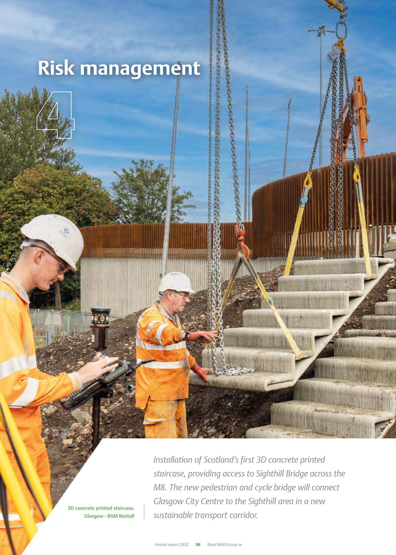
*Installation of Scotland's first 3D concrete printed staircase, providing access to Sighthill Bridge across the M8. The new pedestrian and cycle bridge will connect Glasgow City Centre to the Sighthill area in a new sustainable transport corridor.*
