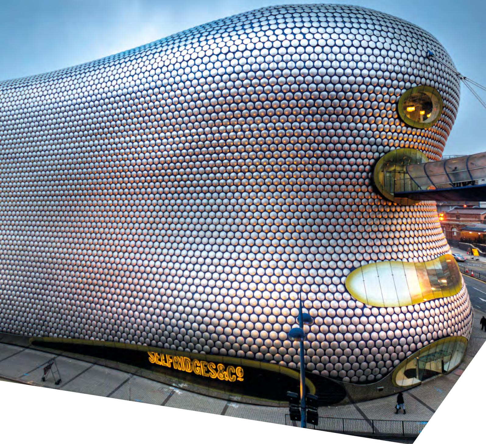
*BAM has removed, cleaned and restored 16,000 aluminium disks while the building's facade was replaced and a new layer of insulation installed.*
