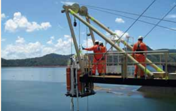
Fugro's specially-engineered launching platform for diving project at the Bento Munhoz da Rocha Netto Hydroelectric dam in Paraná state, Brazil
