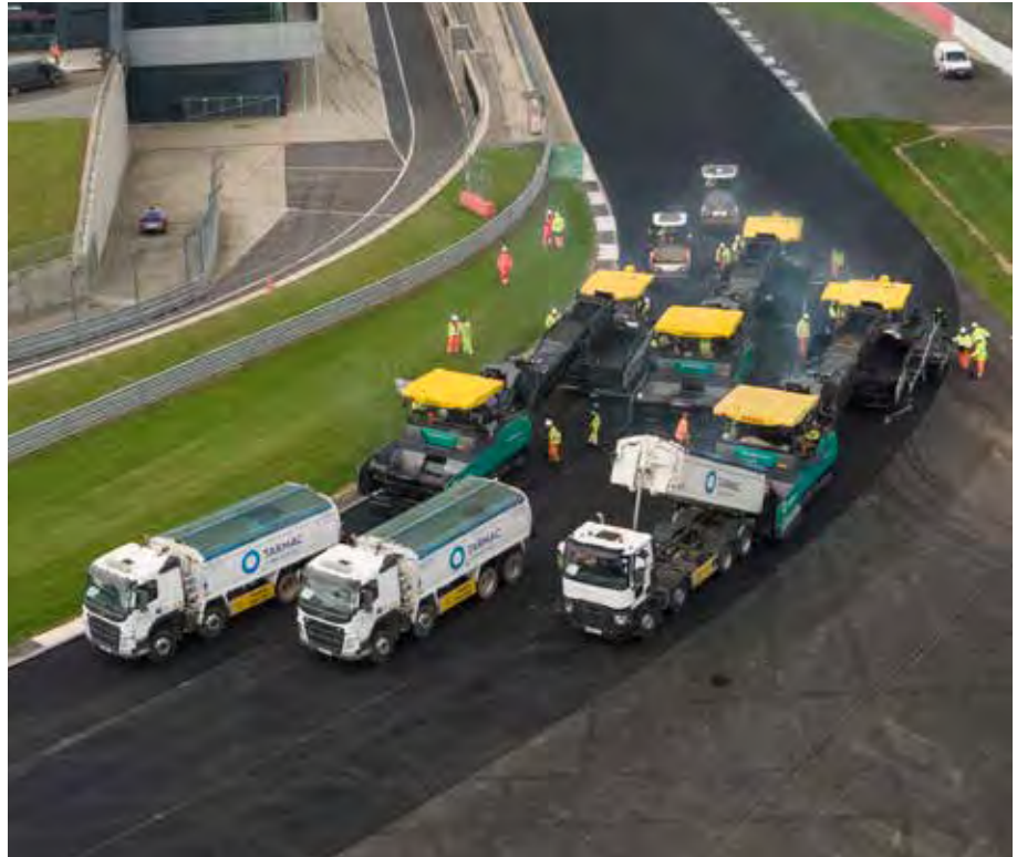
Tarmac, part of CRH's Europe Materials Division, was responsible for resurfacing the world-famous racetrack at Silverstone, home of the British Grand Prix, where Lewis Hamilton clinched a record sixth British Grand Prix victory in 2019. The surface was designed specifically to withstand the extremes of braking and cornering generated by high-performance racing cars and motorbikes. Tarmac used cutting-edge technology and processes to complete the project, including the first use of 3D GPS-guided asphalt planing in the UK as well as state-of-the-art BPO ASPHALT management system software.
