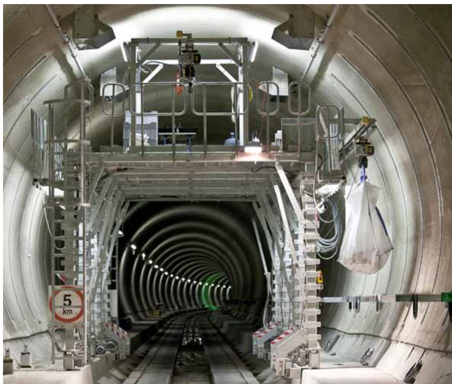
Liefkenshoek railway tunnel (Antwerp) °
