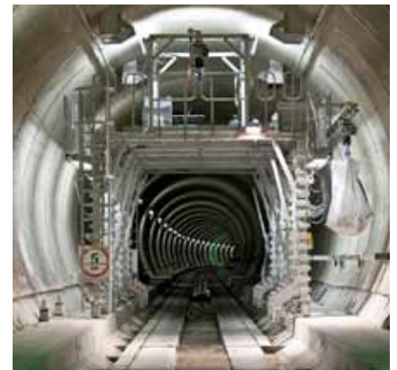
CFE - Liefkenshoek railway tunnel (Antwerp)
