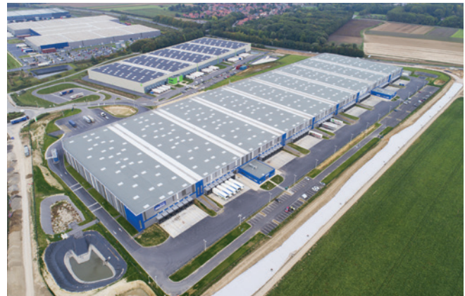
Lauwin-Planque Logistics Centre
