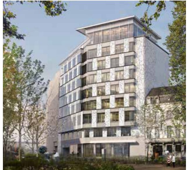
Treesquare Brussels, Belgium
