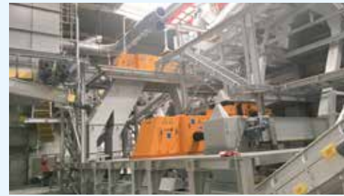
New recycling plant Diksmuide operational
