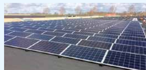
Installation of solar panels at Gits
