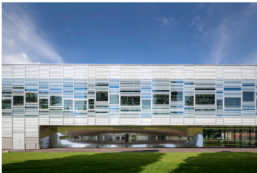
EASE Training Center, Illkirch Graffenstaden - France (European Aseptic & Sterile Environment Training Center) VIB - architecture ballus.viallet © Cyrille Lallement Executed using grade 304 with Uginox Bright surface finish
