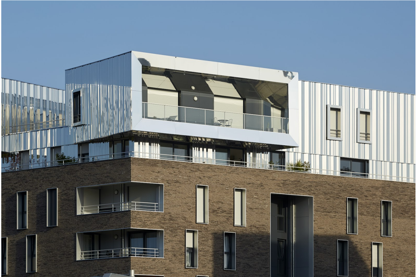
Nova Housing, Strasbourg - France TOA © Frédéric Delangle Executed using grade 304 with Uginox Bright finish
