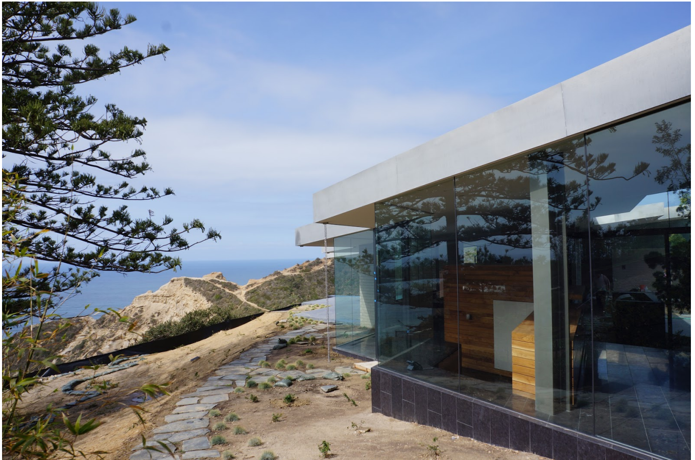
La Jolla, San Diego - USA Architect: Daniel Schmidt © Enduringmetal Executed using grade K44 with Uginox Patina finish
