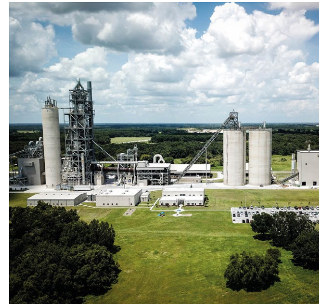
In September 2018, the Board visited Suwannee American Cement Company's Sumterville Plant in Florida. The company, which is part of CRH's Americas Materials Division, has two plants in Florida and is a leading cement supplier in the State. Following the acquisition of Ash Grove in 2018, CRH is now one of the leading cement producers in North America.
