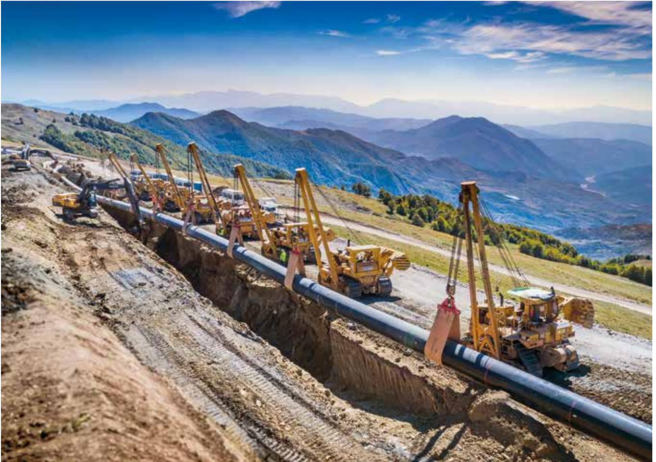
Entrepose is building three onshore gas pipeline sections of the Trans Adriatic Pipeline project. In 2018, its specialist subsidiary Spiecapag finished laying 185 km of gas pipelines in Greece and continued work on two sections with a combined length of 215 km in Albania.
