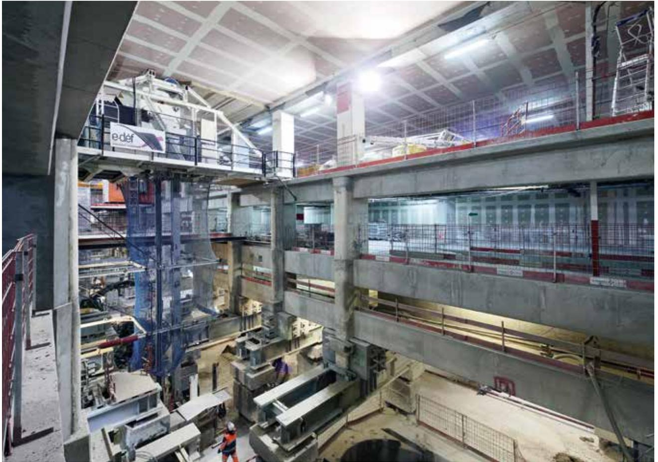
The RER Line E extension west of Paris (Eole programme) is one of the major transport infrastructure projects designed to improve mobility in the Greater Paris area. It includes construction of three new stations. Pictured here, the La Défense station being built at a depth of 35 metres directly under the CNIT convention and shopping centre. The project required installation of temporary structures to support the building.
