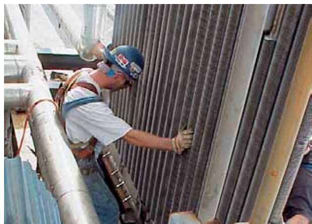
Deltak worker installing a heat recovery steam generator
