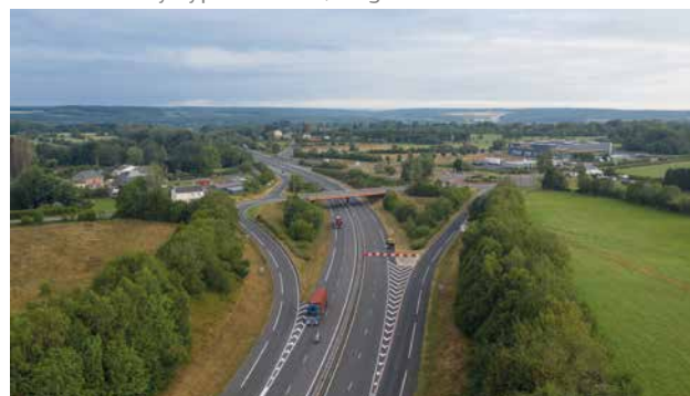
New motorway bypass Couvin, Belgium.
