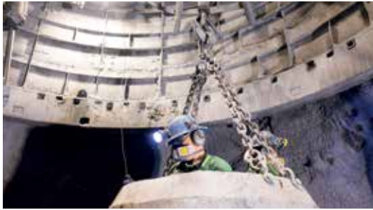
Deepening the Jarillas shaft at Saucito
