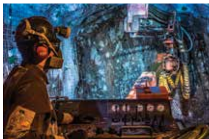
A jumbo drill at work underground
