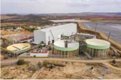
Pyrites plant construction at Fresnillo
