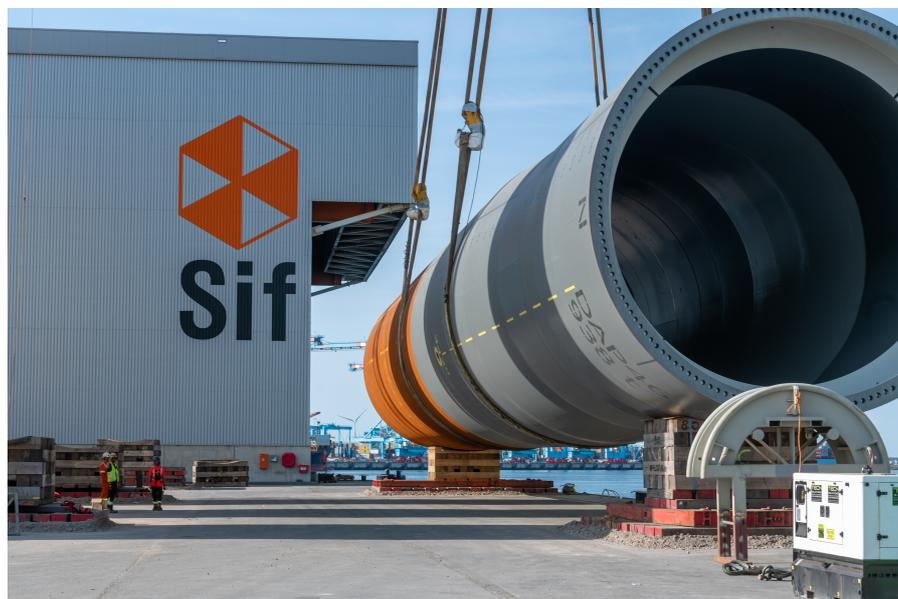
Picture: load-out monopiles for Dogger bank
