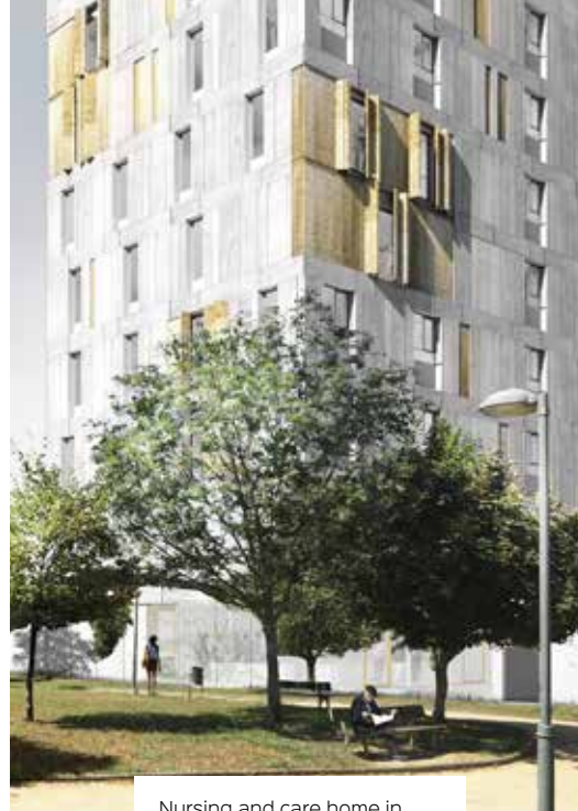
Nursing and care home in construction - Vigo (ES)
