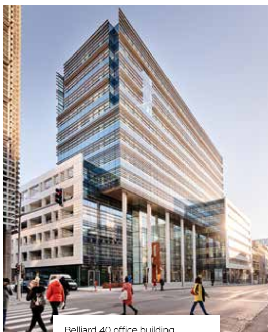
Belliard 40 office building - Brussels CBD (BE)
