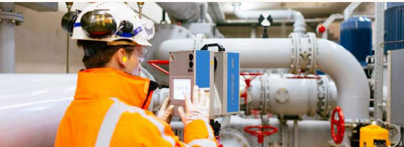
3D laser scanning at water pumping station, Terwisscha, The Netherlands.
