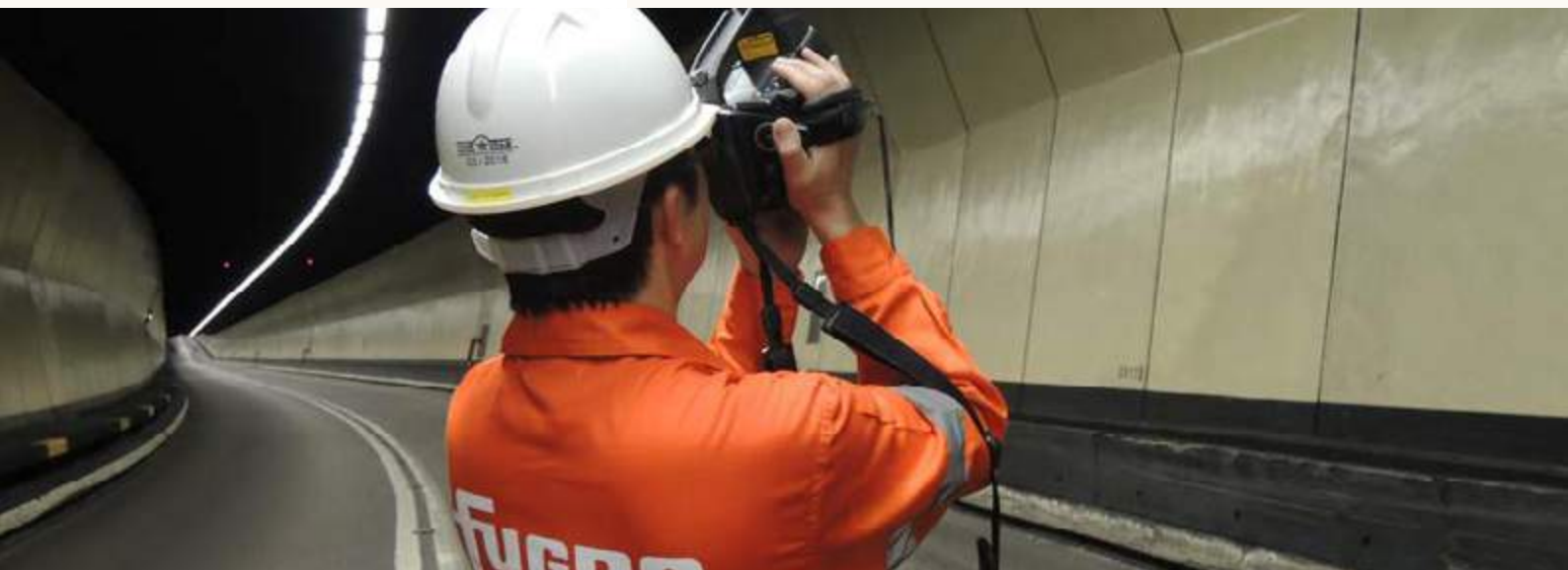
Detecting possible defects in tunnel structure by infrared thermography, Hunghom Cross Harbour Tunnel, Hongkong.
