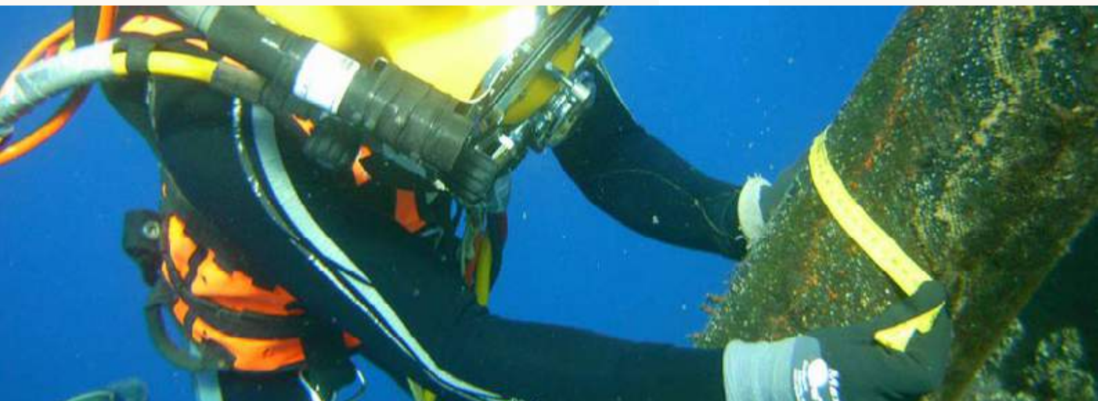
Diver performing inspection, repair and maintenance services.
