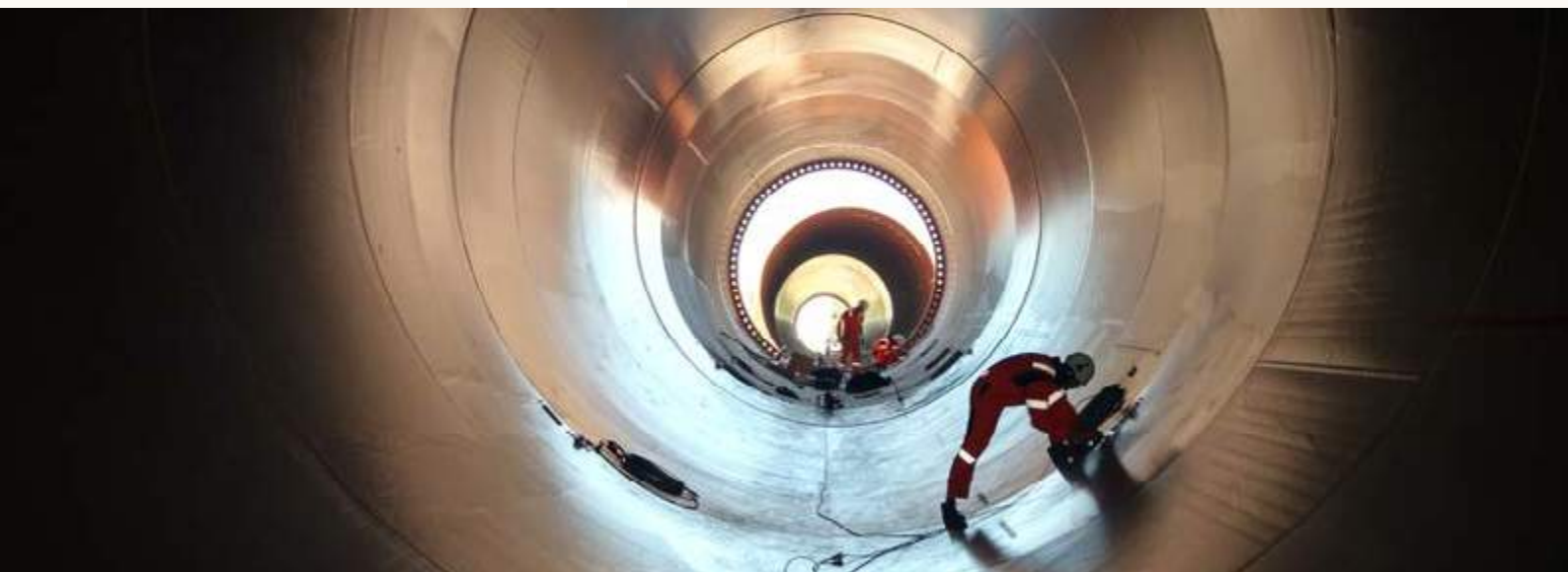
Instrumentation of offshore windfarm monopile for strain, temperature and vibration with fiber optic sensors, Vlissingen, The Netherlands.
