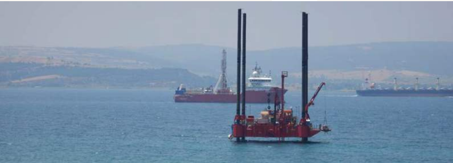
Land and marine site characterisation programme for '1915 Canakkale Bridge', Turkey.
