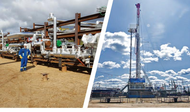
**Innovative well pad design** – We've implemented a sleek new well pad design at our oil sands operations that requires less infrastructure. The new well pads, like this one at Christina Lake, start with the most basic equipment required for safe and reliable operation and have the ability to add infrastructure as required throughout the different phases of the pad lifecycle. This new design significantly reduces both the cost and environmental footprint of our well pads.
