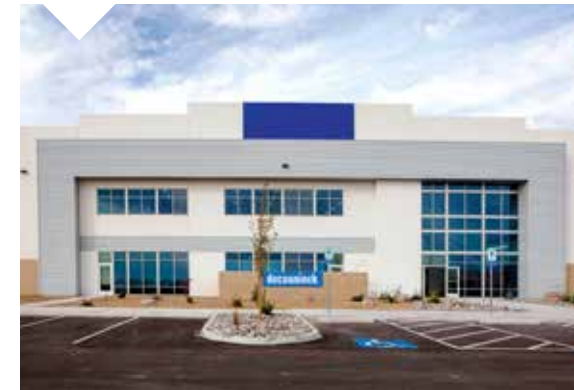
Fernley plant fully operational 24/7 and servicing customers in Western US.
