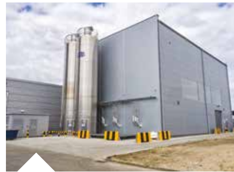
Start compounding in Jasin (Poland).
