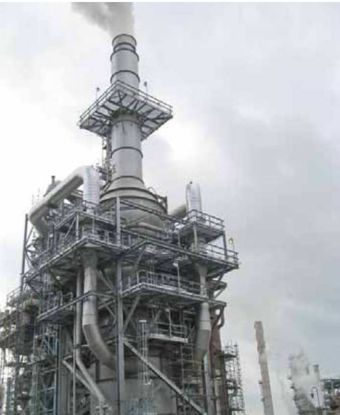
From left to right: Wet gas scrubber built in a U.S. refinery Heat recuperator built by TTC (USA)
