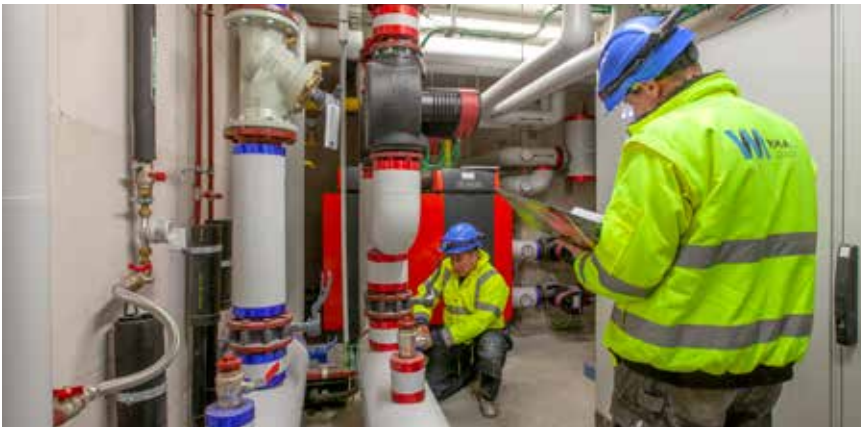
HVAC activities executed by VMA Druart
