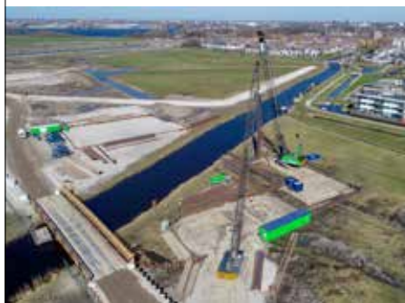
A24 Blankenburgverbinding - The Netherlands
