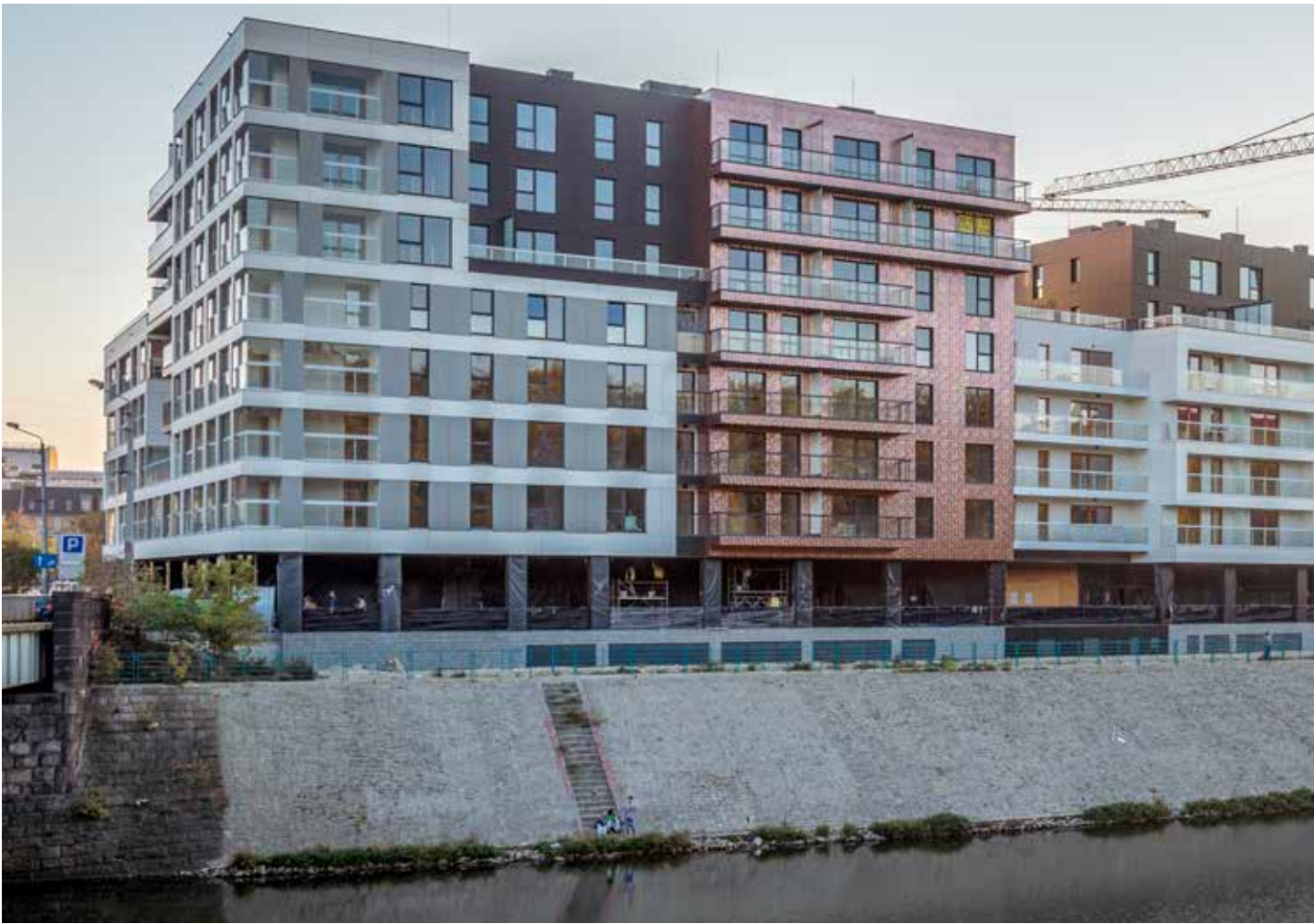
Phase 1 of the Bulwary Ksiazece project - Wrocław
