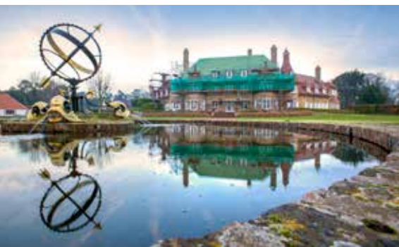
Restoration works - Golfclub Knokke
