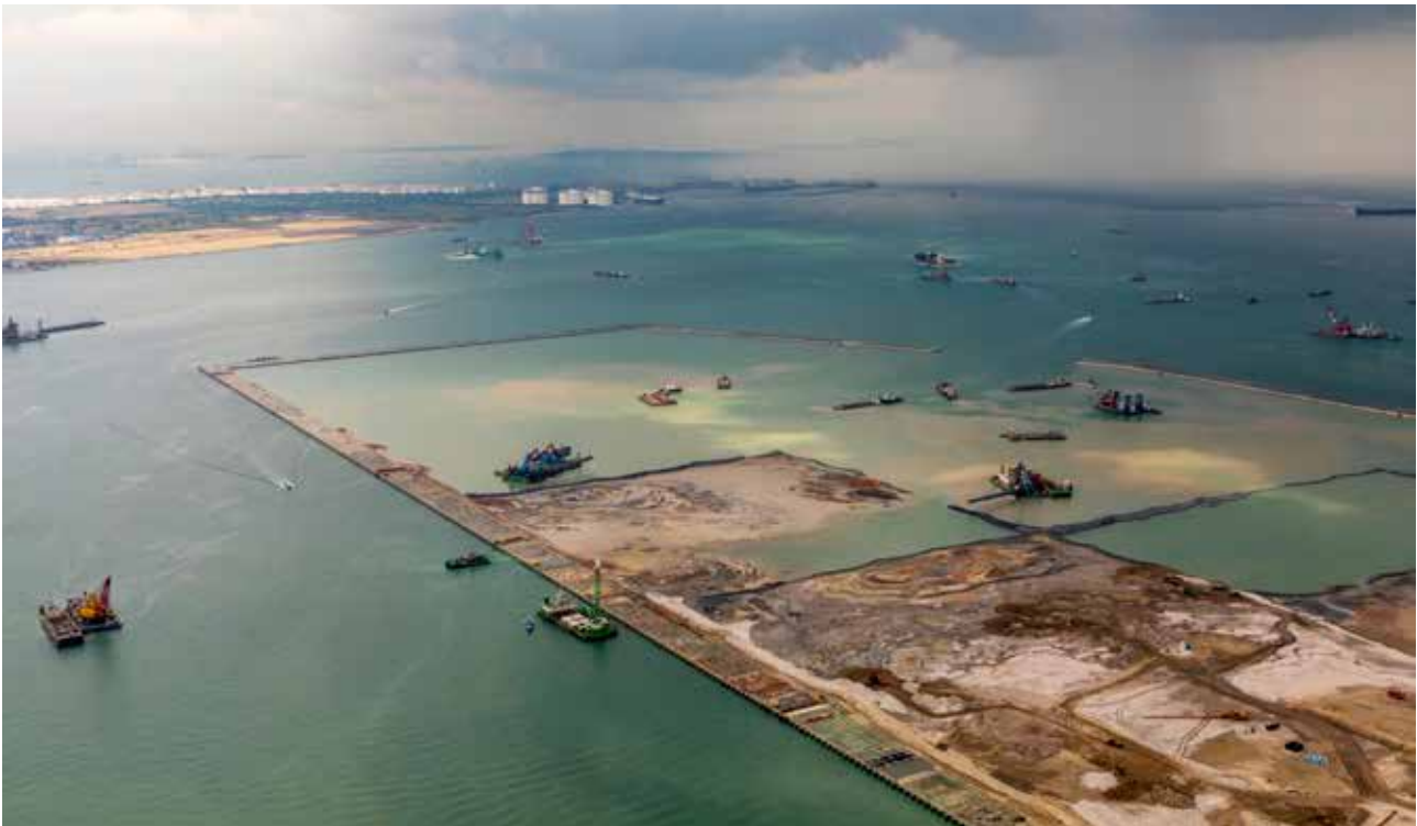
Tuas Terminal Phase 1 (TTP1) - Singapore
