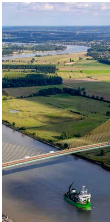
Deepening works of the River Seine - France
