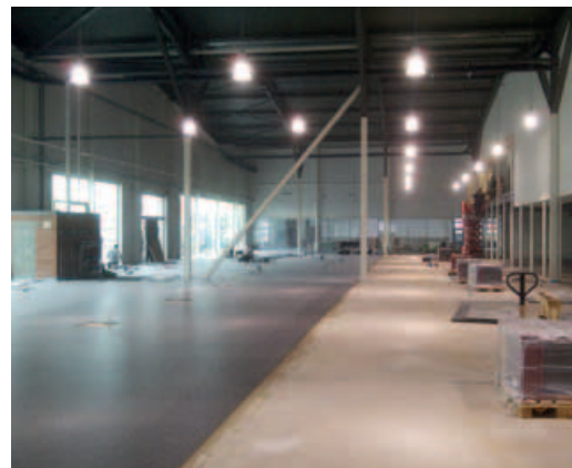
12. placement floor tiles in showroom - finishing offices
