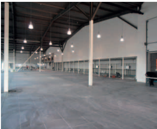
13. installation of building techniques
