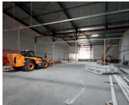
14. positioning cable ducts in workshop
