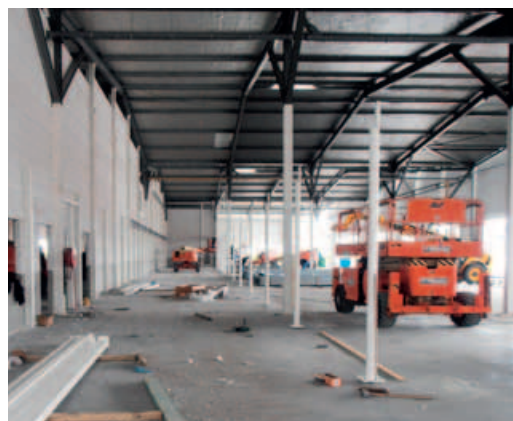
8. erection fire proof wall between workshop and showroom
