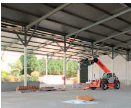
3. erection of fire proof wall connecting adjacent areas
