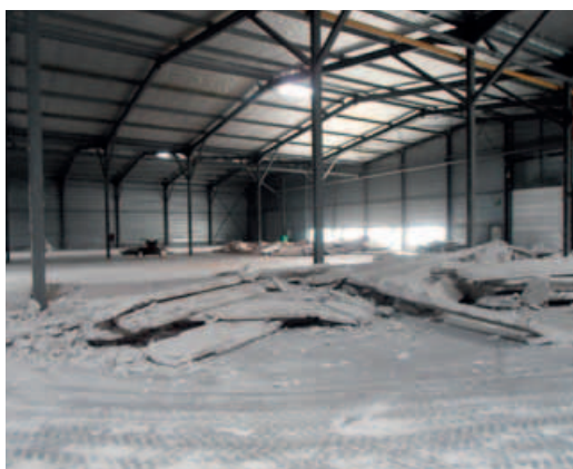
1. demolishing of existing walls
