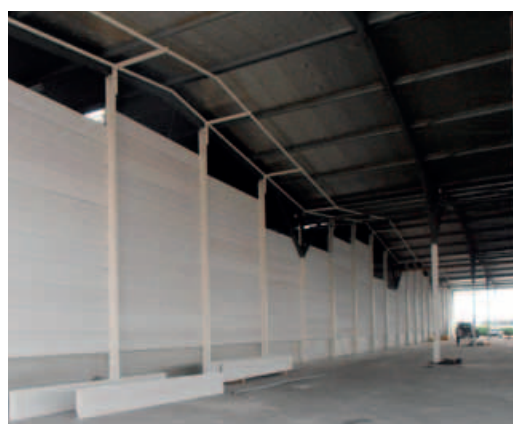
4. construction of flashover security element
