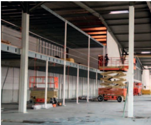
9. installation support structure for first floor offices
