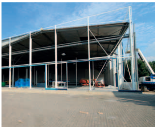
5. installation support structure for new facade cladding
