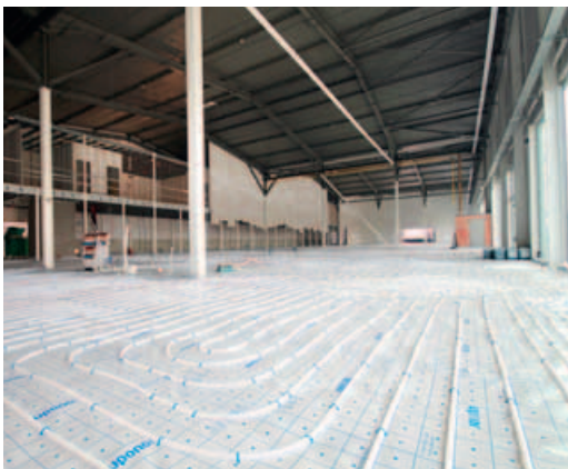
11. installation under floor heating system in showroom
