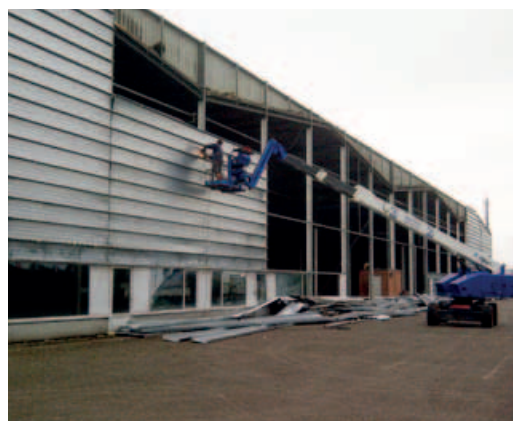
2. removal existing facade cladding
