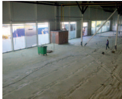
10. spraying of floor insulation in showroom
