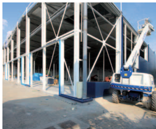
6. placing of sandwich panels new facade
