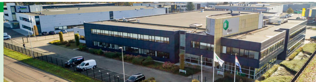
Meco Equipment Engineers office, Drunen, the Netherlands.
