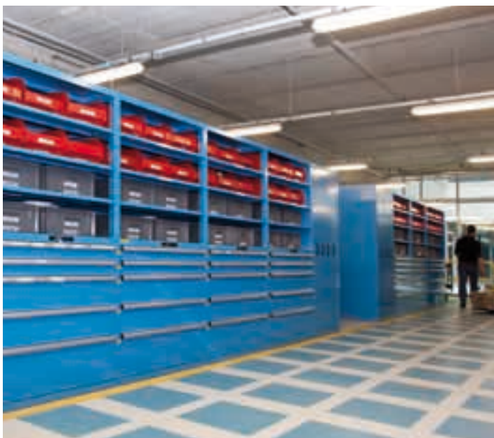
In the H6 hangar, an inventory of components and tools <<<
