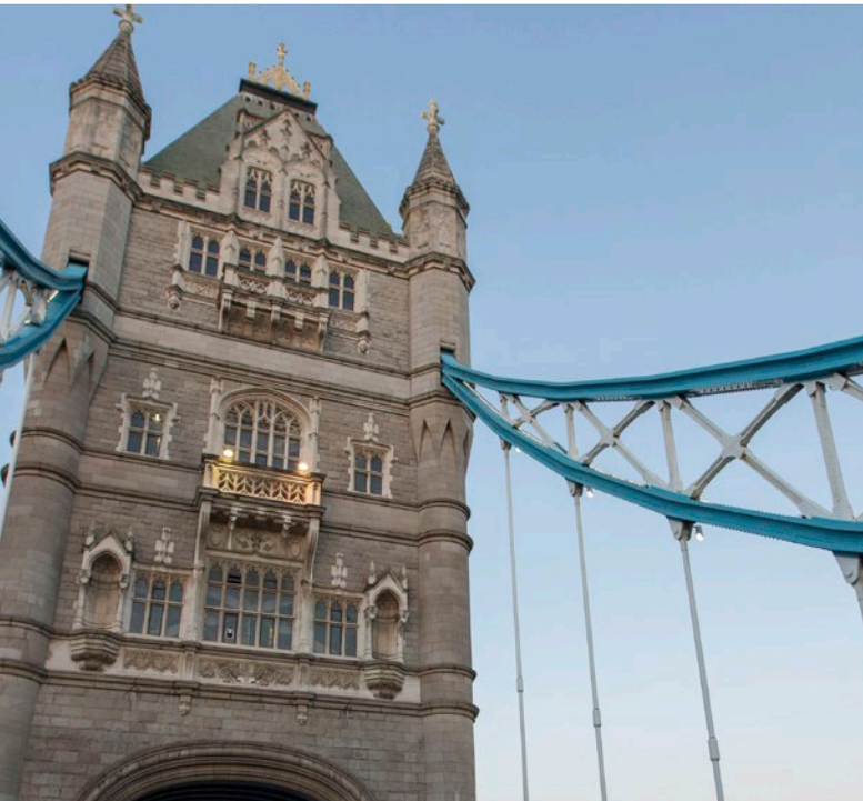
Repair and maintenance of the Tower Bridge, London. BAM Nuttall.
