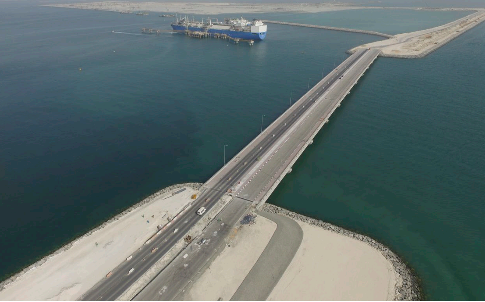
Construction of Dubai's Jebel Ali Port in the United Arab Emirates. Construction of 2,240 metres of quay wall, 2,240 metres of land side crane beam to accommodate 100-tonne STS cranes as well as a 440-metres long access bridge and a 2.6-kilometres causeway to link the new terminal being built on an island of reclaimed land to the main port. BAM International, BAM Infraconsult.
