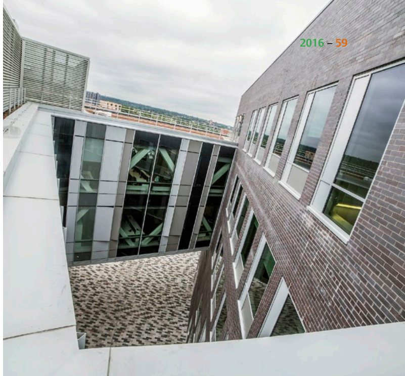
Adelphi Arts Centre, University of Salford. BAM Construct UK.
