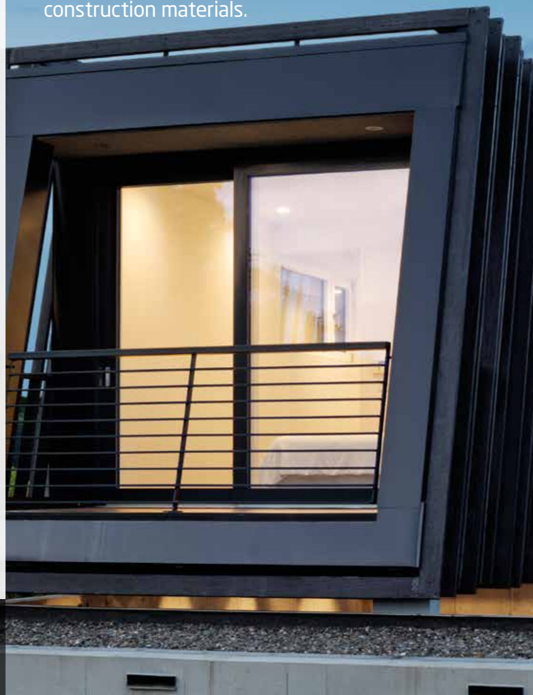
Delta Millworks used our sustainable product Accoya® to manufacture the siding for this unique home in New York state. Using a Japanese finishing technique called 'shou sugi ban' the Accoya® was charred to give the house's façade a modern, weathered texture.
