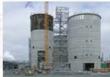
The wood chip silos nearing completion at the Hull Tricoya® plant
