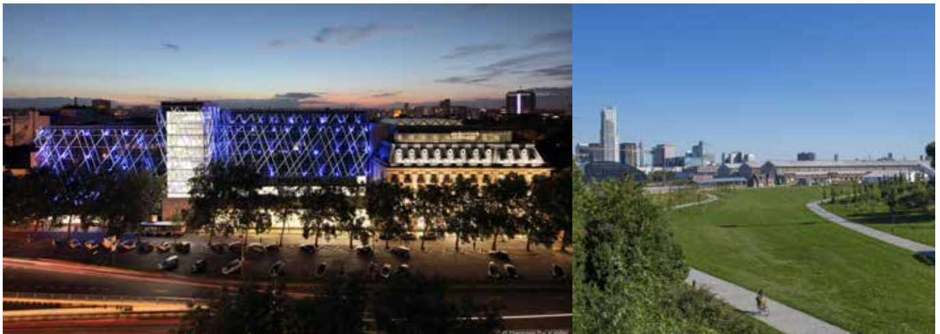
CFE - The headquarters of AXA obtained BREEAM Excellent and the sustainability certificate Passive 2015
