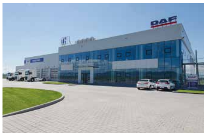
New garage in Sofia - Bulgaria
