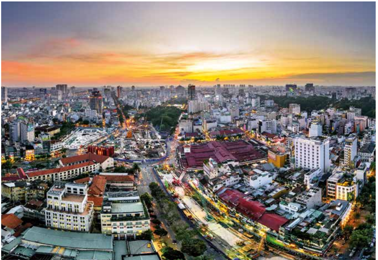
Diaphragm wall works at the worksite for Line 1 of the Bến Thành - Suối Tiên metro in Ho Chi Minh City, Vietnam, the country's first metro system.
