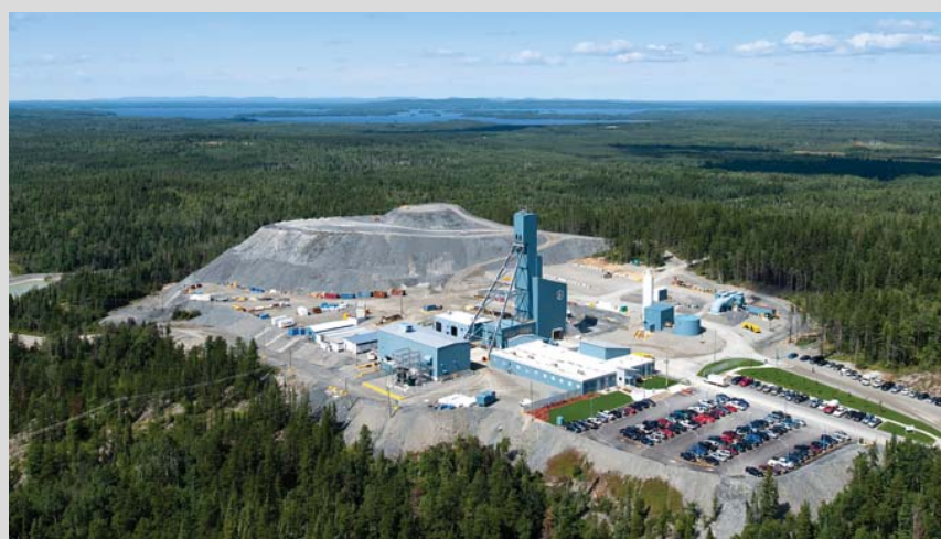
Once production from Lapa mine is completed later in 2018, official reclamation and restoration work will begin, with full closure anticipated in 2026–2027.
