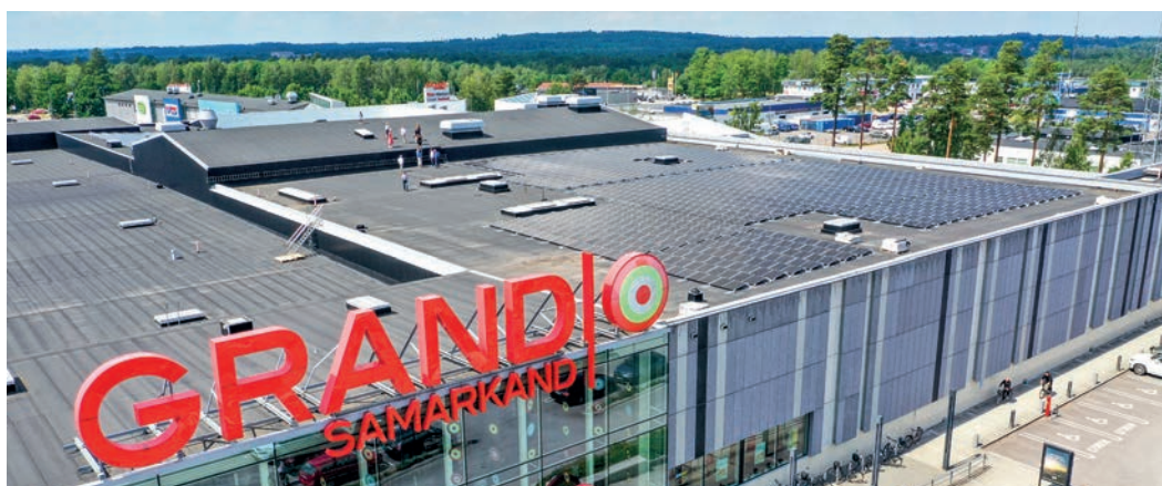
Solar panel roof installation at Grand Samarkand.
