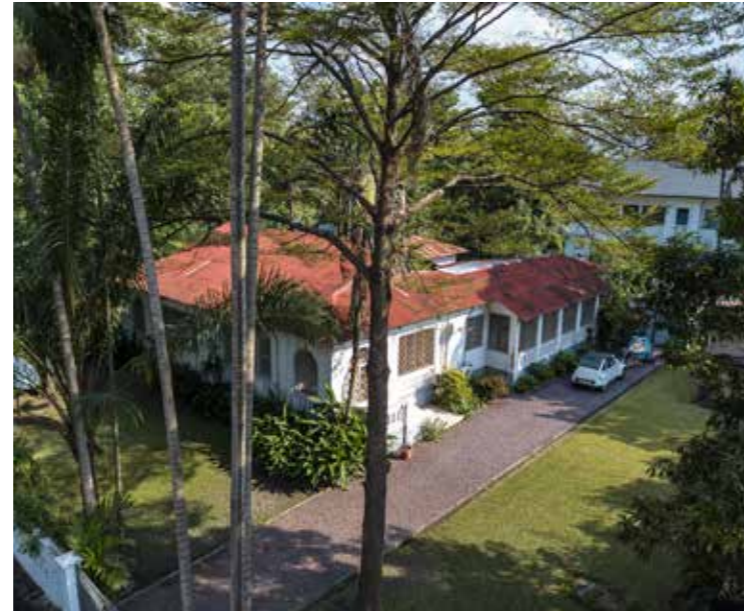
Villa in the historical compound.
