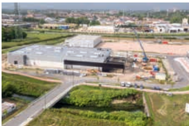
Building site of D'leteren's new multi-brand bodywork in Drogenbos, near Brussels.
