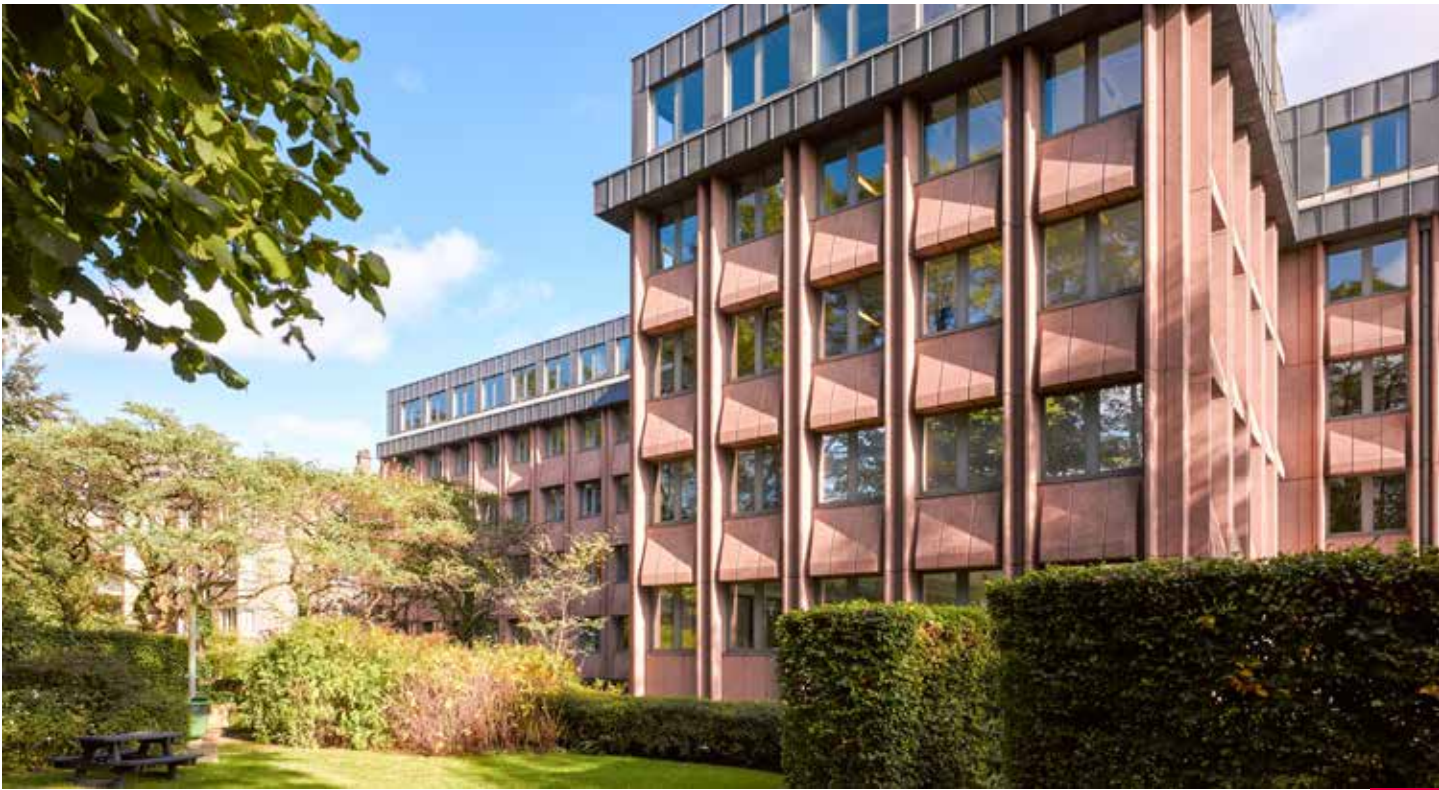
Office building - Souverain 280 - Brussels (BE)
