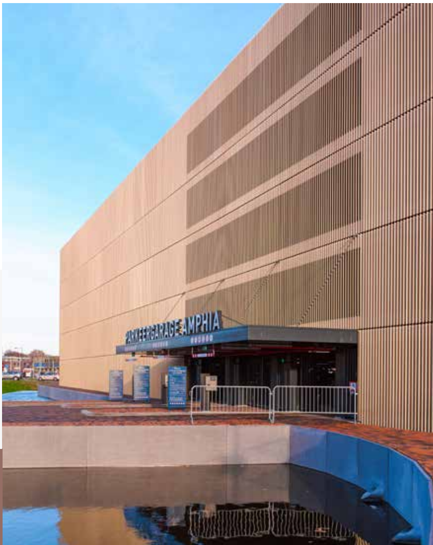
Parking building of the hospital Amphia Breda (NL)
