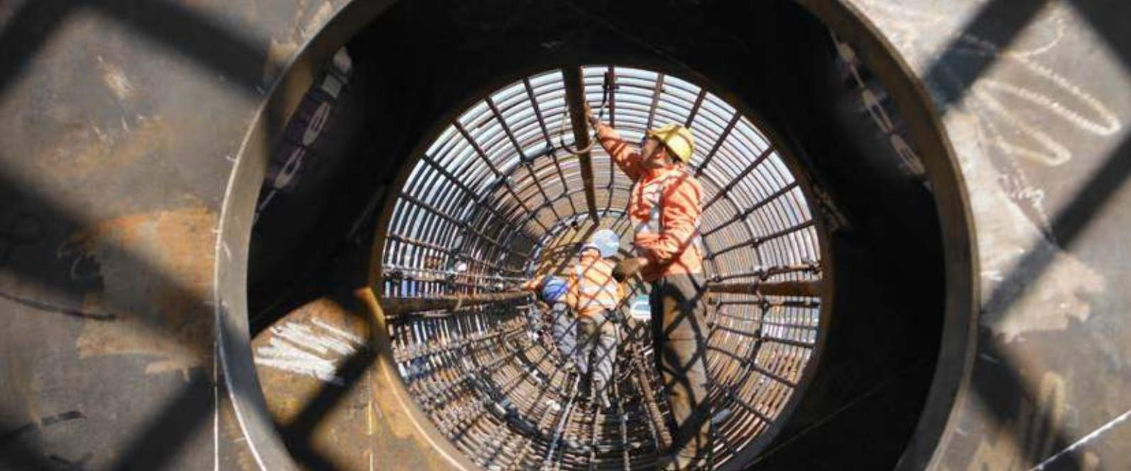
Installation of instruments for Osterberg Cell load test, Lantau, Hong Kong.
