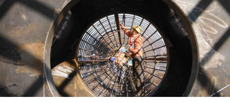
Installation of instruments for Osterberg Cell load test, Lantau, Hong Kong.
