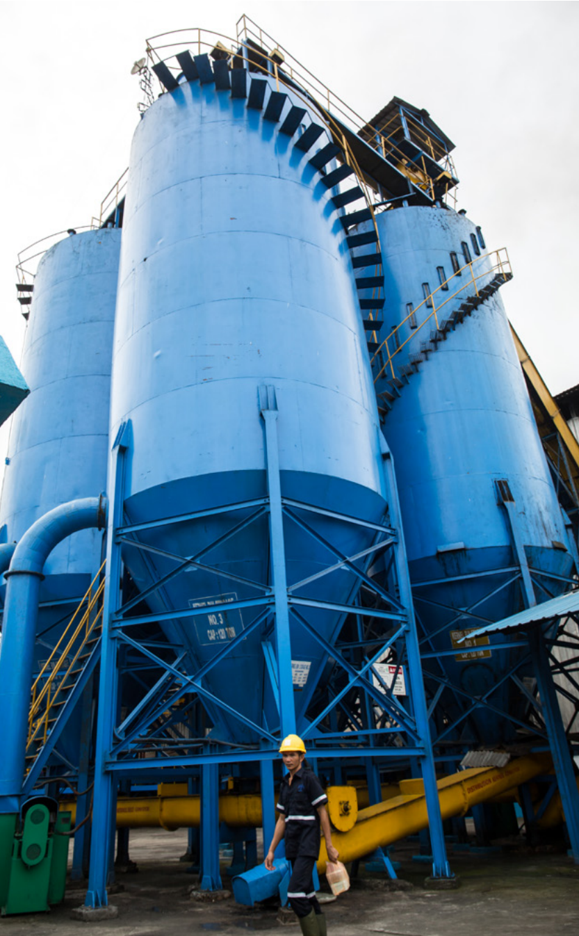
Silos for bulk storage of palm kernels
