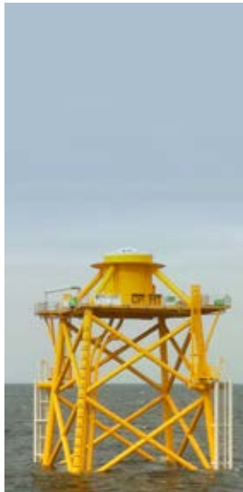
components for jackets for offshore wind turbines and substations
