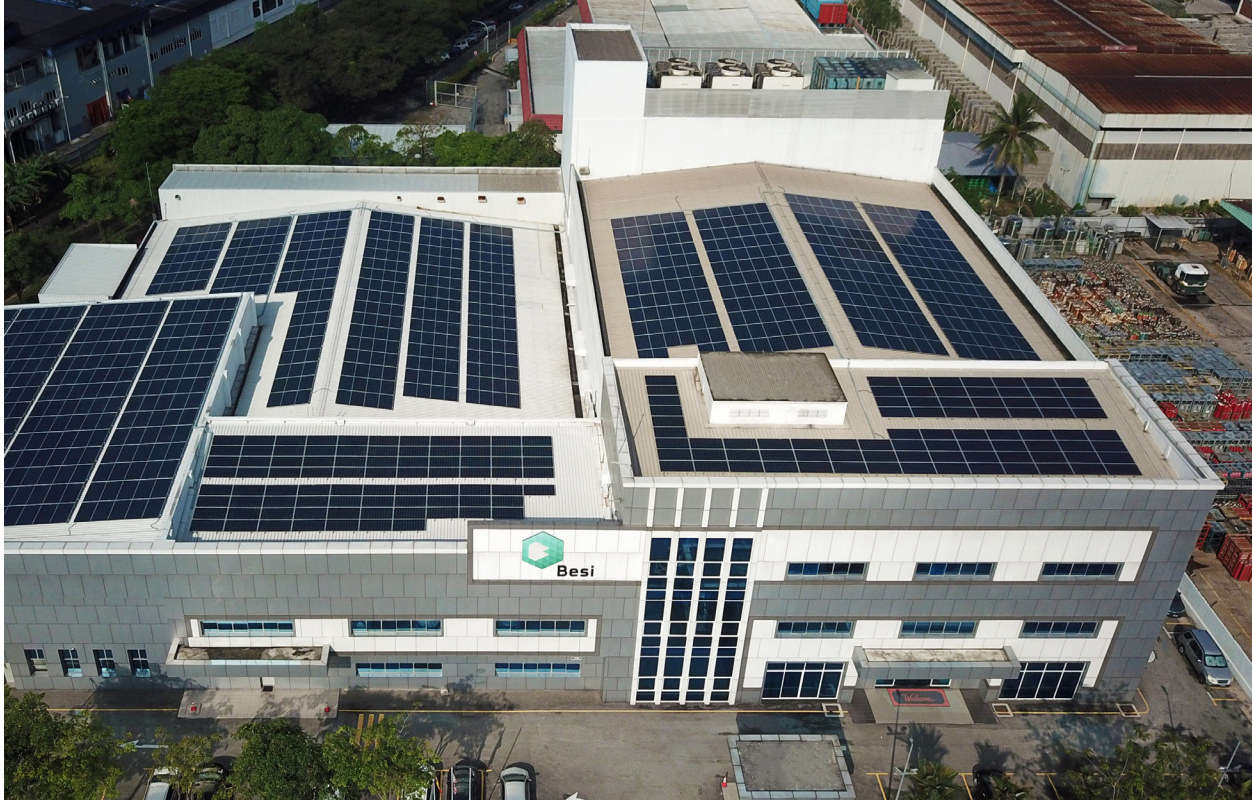
Solar panels installed at Besi APac, Malaysia.
