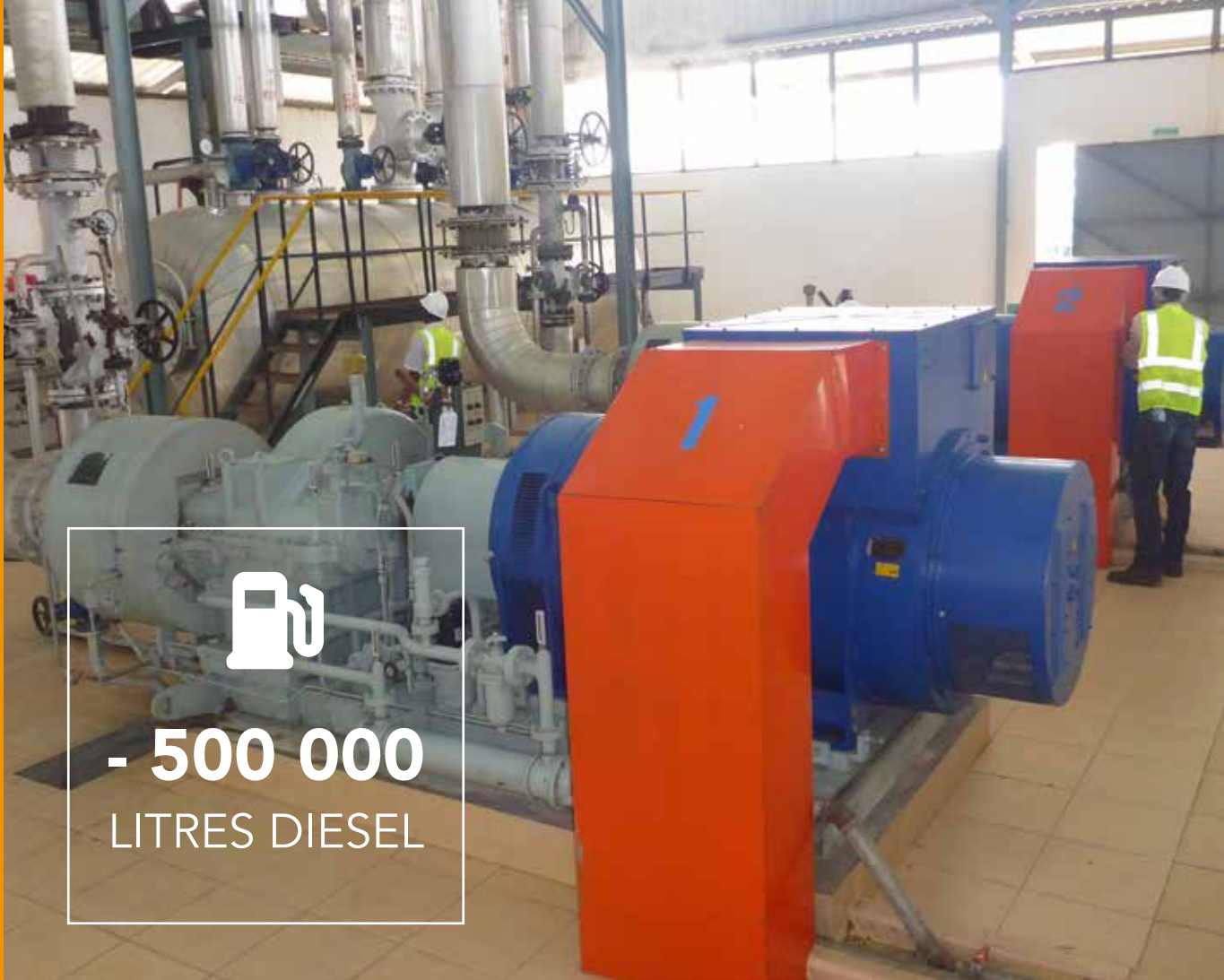
Two steam turbines in the foreground, and the steam expansion tank in the background
