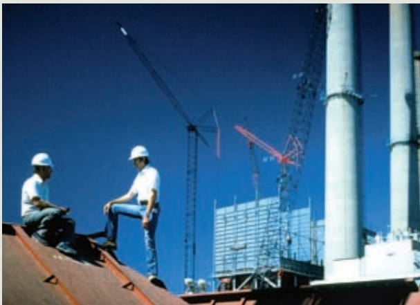
Workers on construction site
