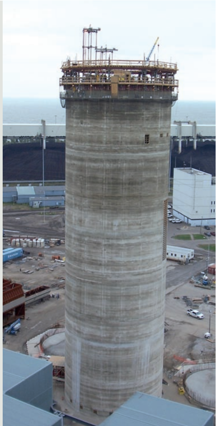
Concrete chimney for a power plant in Southern USA
