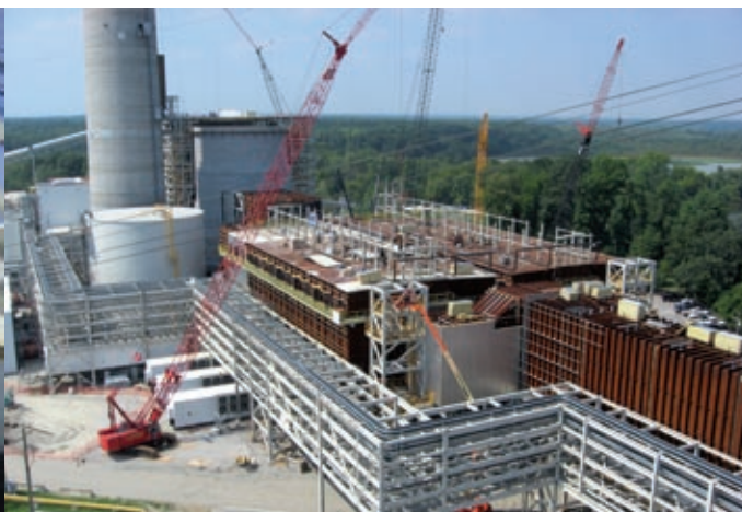
Fabric filter for a power plant in Virginia, USA
