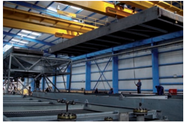
Production of air cooler bundles in the new plant in Saudi Arabia
