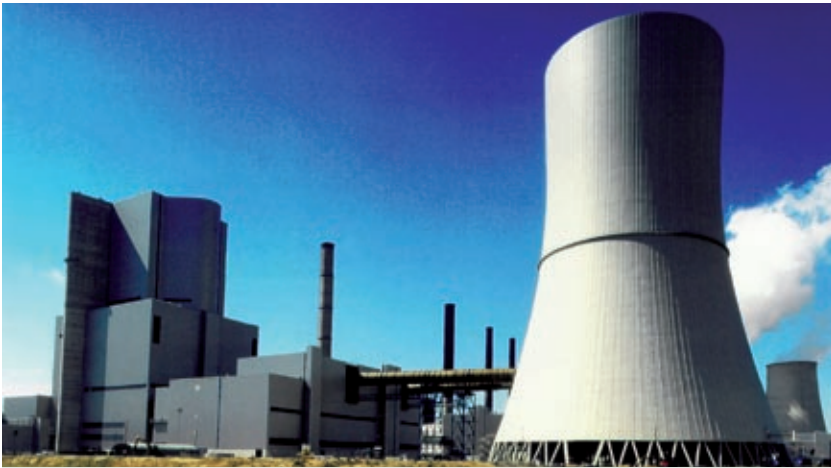
Natural draft cooling tower with flue gas injection, Germany
