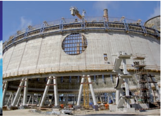
Erection of a natural draft cooling tower in Lagisza, Poland
