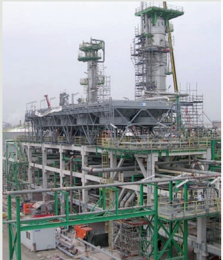
General view of a refinery and its air coolers
