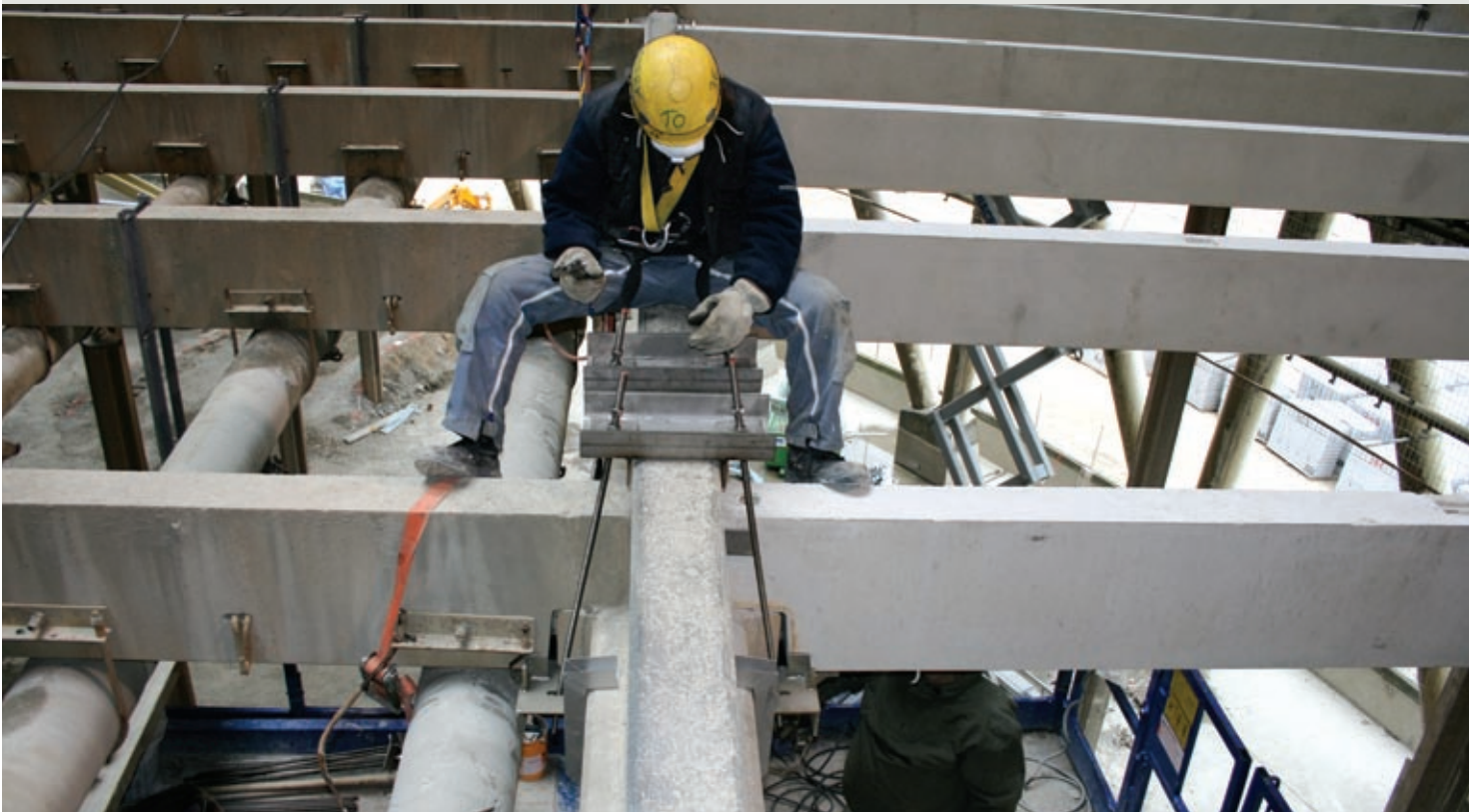
Work on a cooling tower in France
