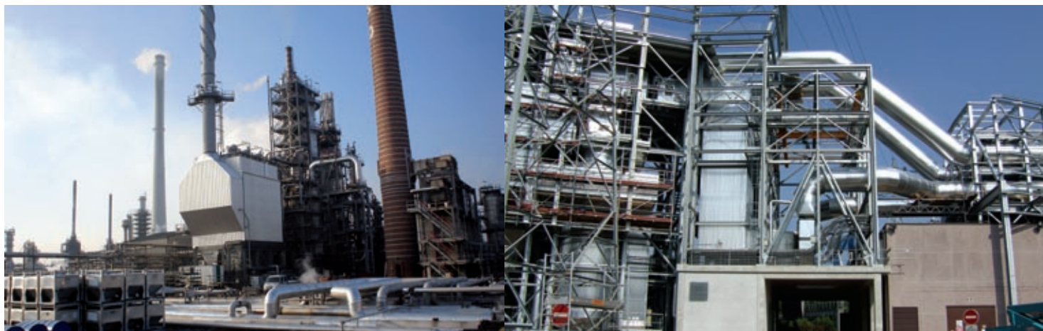
Electrostatic precipitator installed in an oil refinery, Antwerp, Belgium
