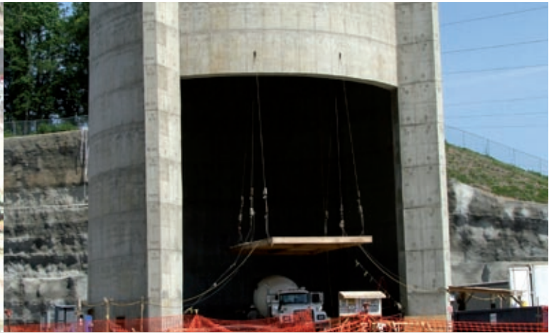
Erection of a concrete chimney in USA (detail of lower part)
