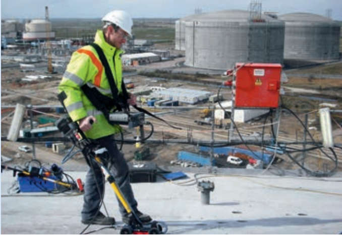
Ground Penetrating Radar survey on concrete LNG tank, United Kingdom.
