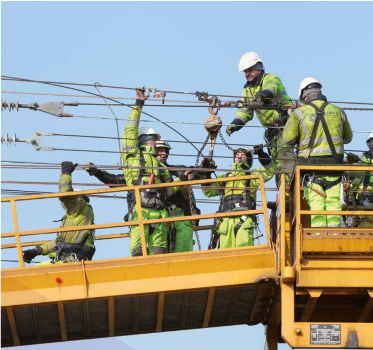
↑ Adjustment works overhead lines Brugge
