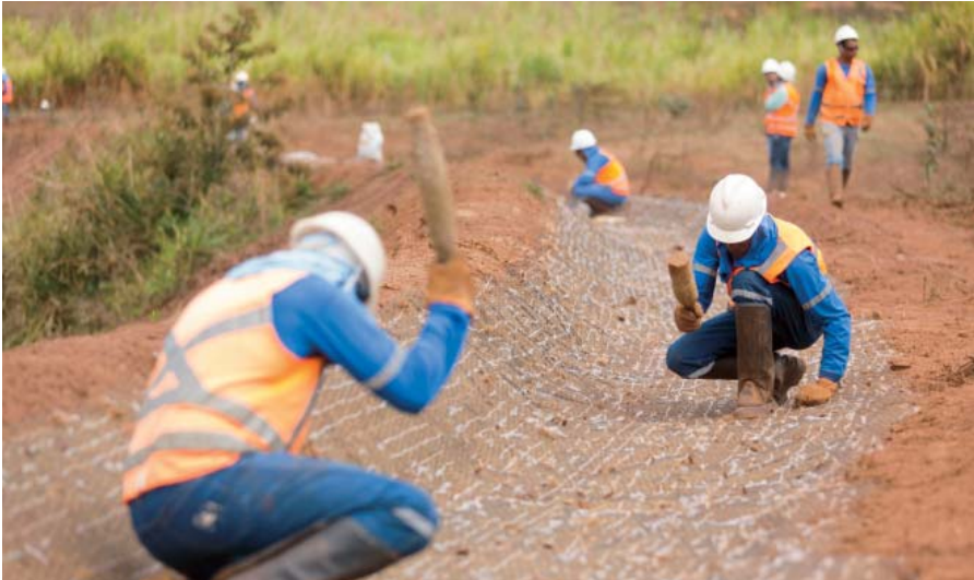
Erosion control measures at Rio Doce floodplains.
