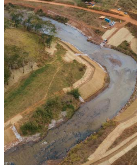
River stabilisation works on the Gualaxo do Norte River.
