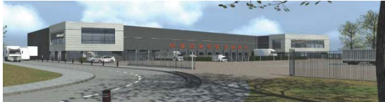
Montea «Space for Growth» - site Schiphol Logistics Park (NL)
