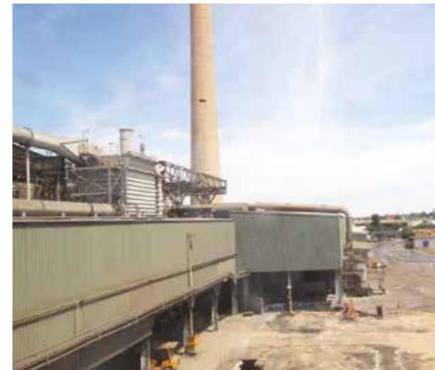
BEFORE INSTALLATION OF THE TSL FURNACE AT PORT PIRIE (Q1 2015)
