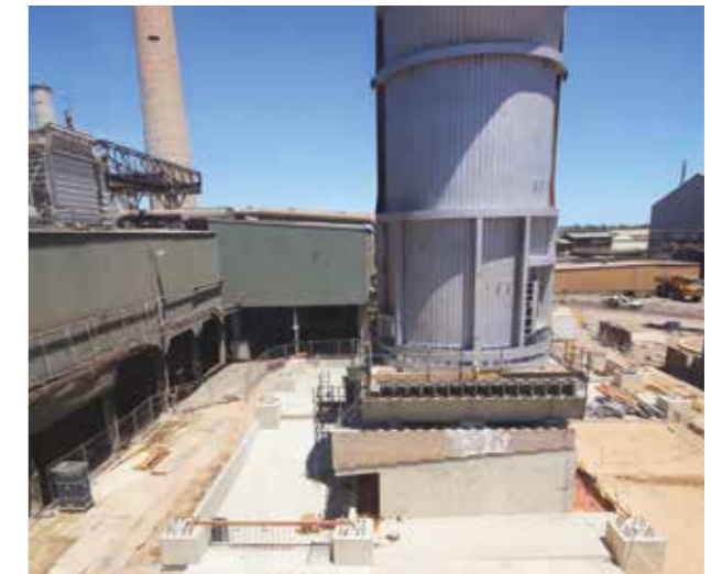
AFTER INSTALLATION OF THE TSL FURNACE IN PORT PIRIE (Q1 2016)
