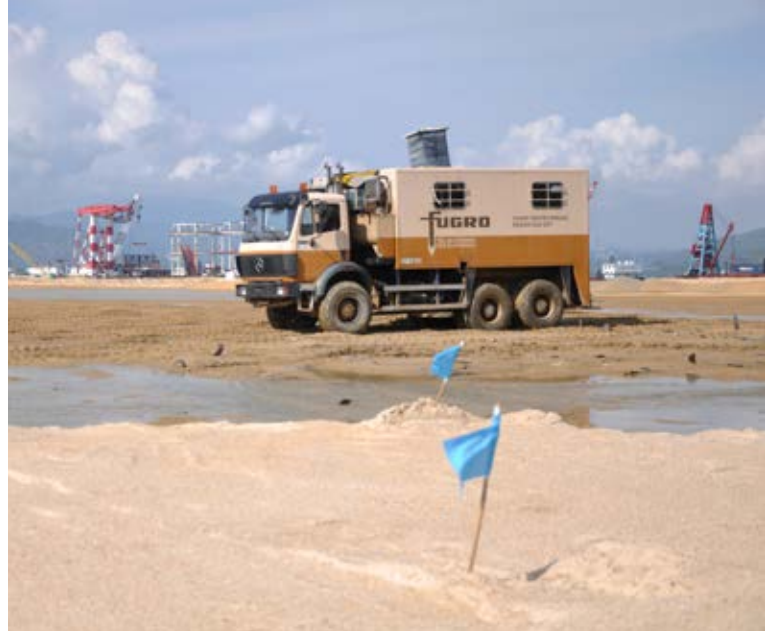
CPT testing of land reclamation in Hong Kong.
