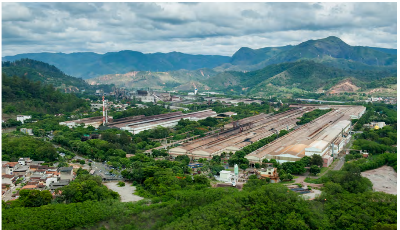
Aperam Stainless & Electrical - Timóteo plant
