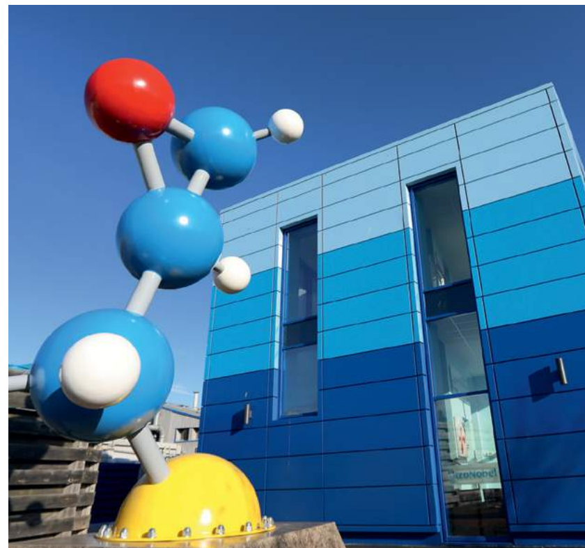
Early in the year, we officially opened a new €13 million R&D innovation campus at our Felling site in the UK. The lab complex enables our technical experts to test products for the marine, oil and gas industries in conditions that mimic the world's most extreme environments.
